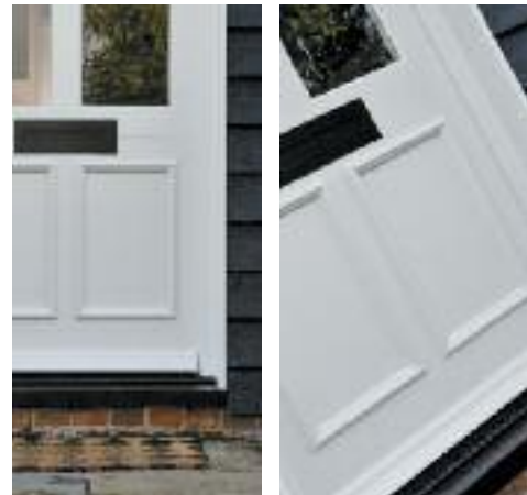
Flat panel with Putty Bolection Moulding – Listed Range
