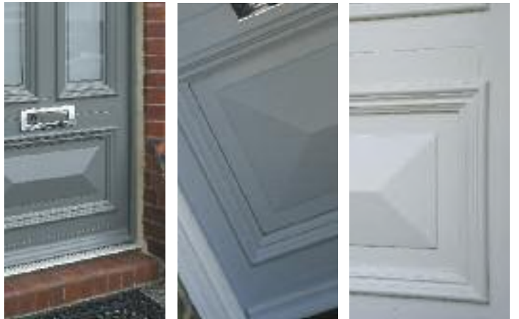
Envelope panel with Bolection Moulding
