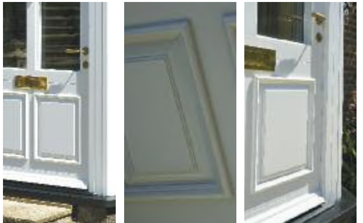
Raised and Fielded with Putty Bolection Moulding – Listed Range
