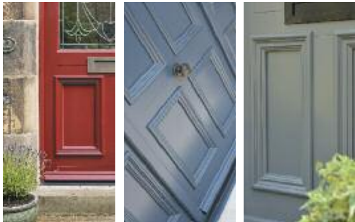
Flat Panel with Bolection Moulding
