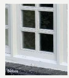
Deco casement windows finished in 'French Grey', with 18mm astragal glazing bars and manufactured in Engineered Meranti Hardwood.
