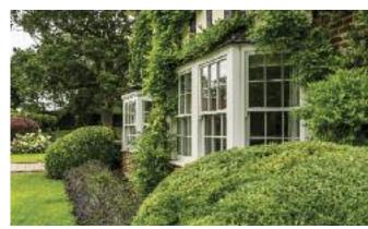
Slim sash windows, casements and arched French doors in a range of configurations, all in the colour "Smoke Cream" externally with 18mm astragal bars.
