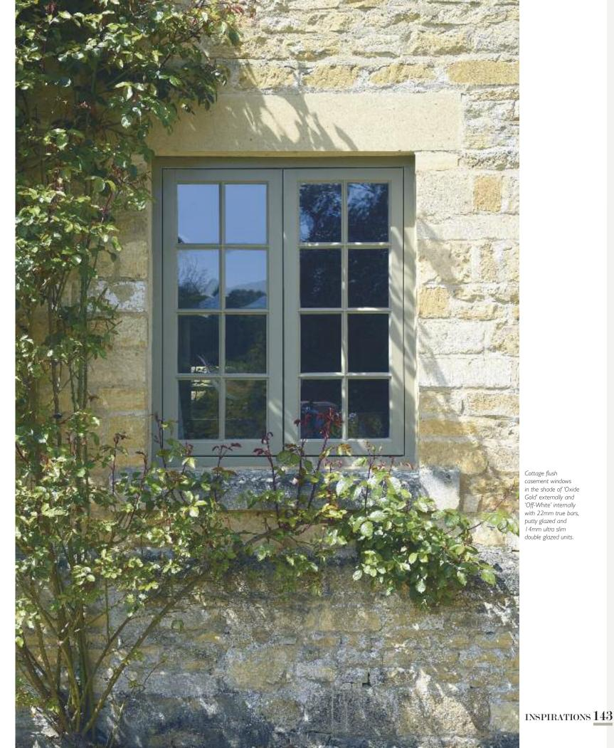
n the shade of 'Oxide Gold' externally and 'Off-White' internally double glazed units.
