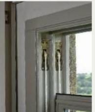
Slim sash windows with traditional cords & weights, finished in a colour complementary to Farrow & Ball 'Hardwick White' with 36mm astragal glazing bars and Mottled Antique Brass hook fasteners and sash lifts.
