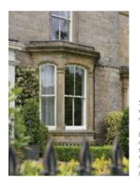
Slim sash windows with chains and weights mechanisms, featuring l 8mm astragal glazing bars, all finished in a colour complementary to Farrow & Ball "All White". Manufactured
