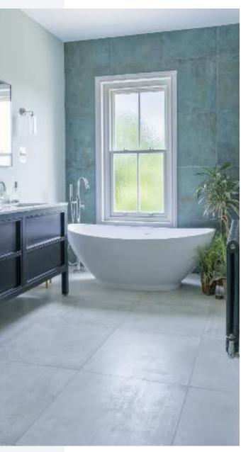
Slim sash windows with hidden spring mechanisms and 18mm astragal glazing bars, finished in "Off-White". Manufactured in Engineered European Redwood.
