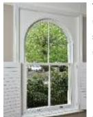
The slim sash windows have swept heads to fit the original openings, featuring krypton gas filled double glazing units for superior thermal and noise insulation.
