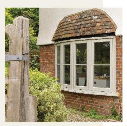
Our timeless flush casement windows and French doors were specified, with 18mm horizontal astragal glazing bars, and a dual colour finish, of 'French Grey' externally and a colour complementary to Farrow & Ball 'Wimborne White' internally.
