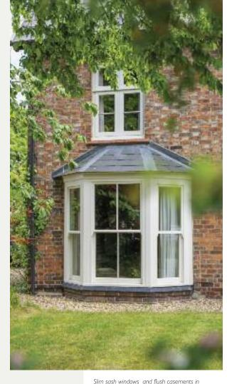
Slim sash windows and flush casements in various styles and configurations, all with 18mm astragal bars and finished in "Cream". Manufactured in Engineered European Redwood.
