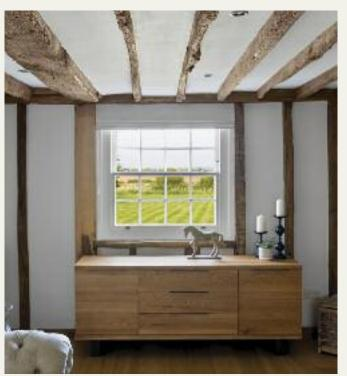
Listed slim sash windows finished in "White", hung on cords and weights, with single glazing, true bars, traditional putty glazed finishing and Oil Rubbed Bronze hardware. Manufactured in Engineered European
