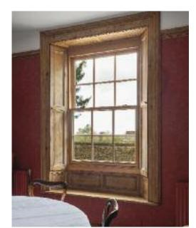
Slim sash windows with 18mm astragal glazing bars, and hung on traditional cords and weights. Finished in a colour complementary to Farrow & Ball "White Tie" externally with some in a "Light Oak" stain internally. Manufactured in Engineered European Redwood.
