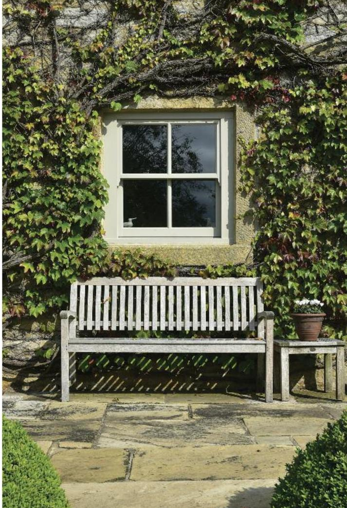
Slim sash windows finished in a colour complementary to Farrow & Ball 'Hardwick White' with decorative sash horns and 36mm astragal glazing bars.
