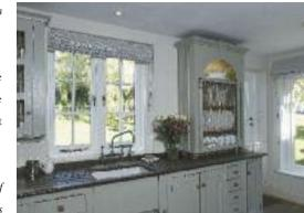
Flush casement windows finished in 'Porcelain' externally and 'White' internally with regular and gothic style 27mm astragal glazing bars and featuring Antique Brass Unlacquered Contour handles and pegstays from Samuel Heath.
