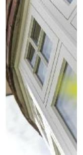
Flush casement windows finished in 'Off-White', with I 8mm astragal glazing bars. Manufactured in Engineered European Redwood.
