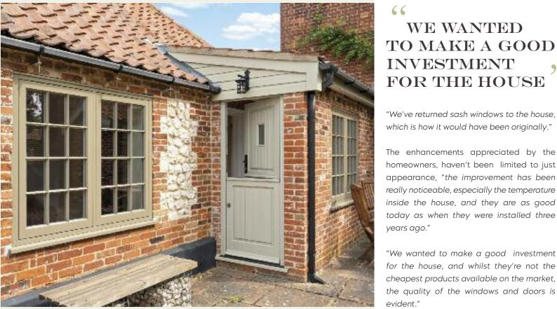
finished in 'Oxford Clay' with I Symm astragal glazing bars and Staverton style stable door finished in 'French Grey' with a Black Avon handle. All manufactured in Engineered European
