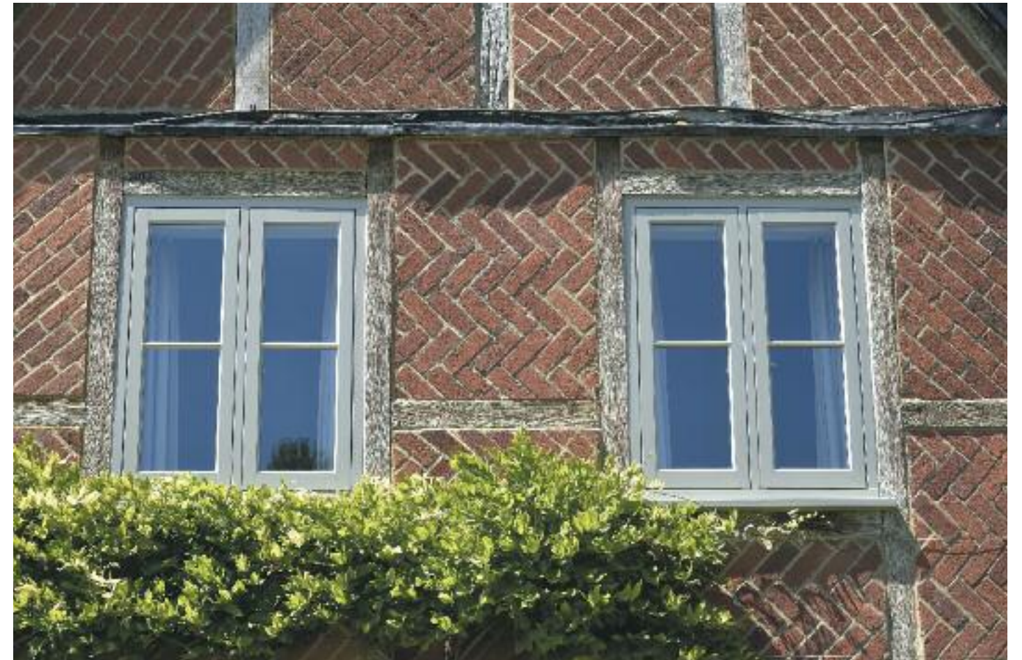
Flush casement windows finished in a colour complementary to Farrow & Ball's 'Hardwick White' externally and 'Ammonite' internally with 24mm true bars, putty glazing and 14mm ultra slim double-glazed units.
