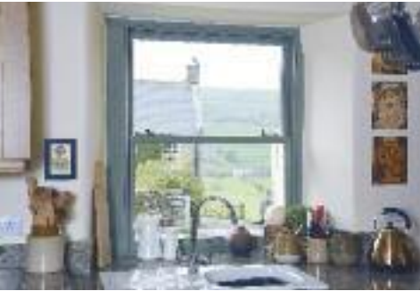
Slim sash windows, flush casements and cottage casements all finished in 'Tent Grey' and manufactured in Engineered Meranti Hardwood featuring 18mm double glazed units and 4mm single glazing also.
