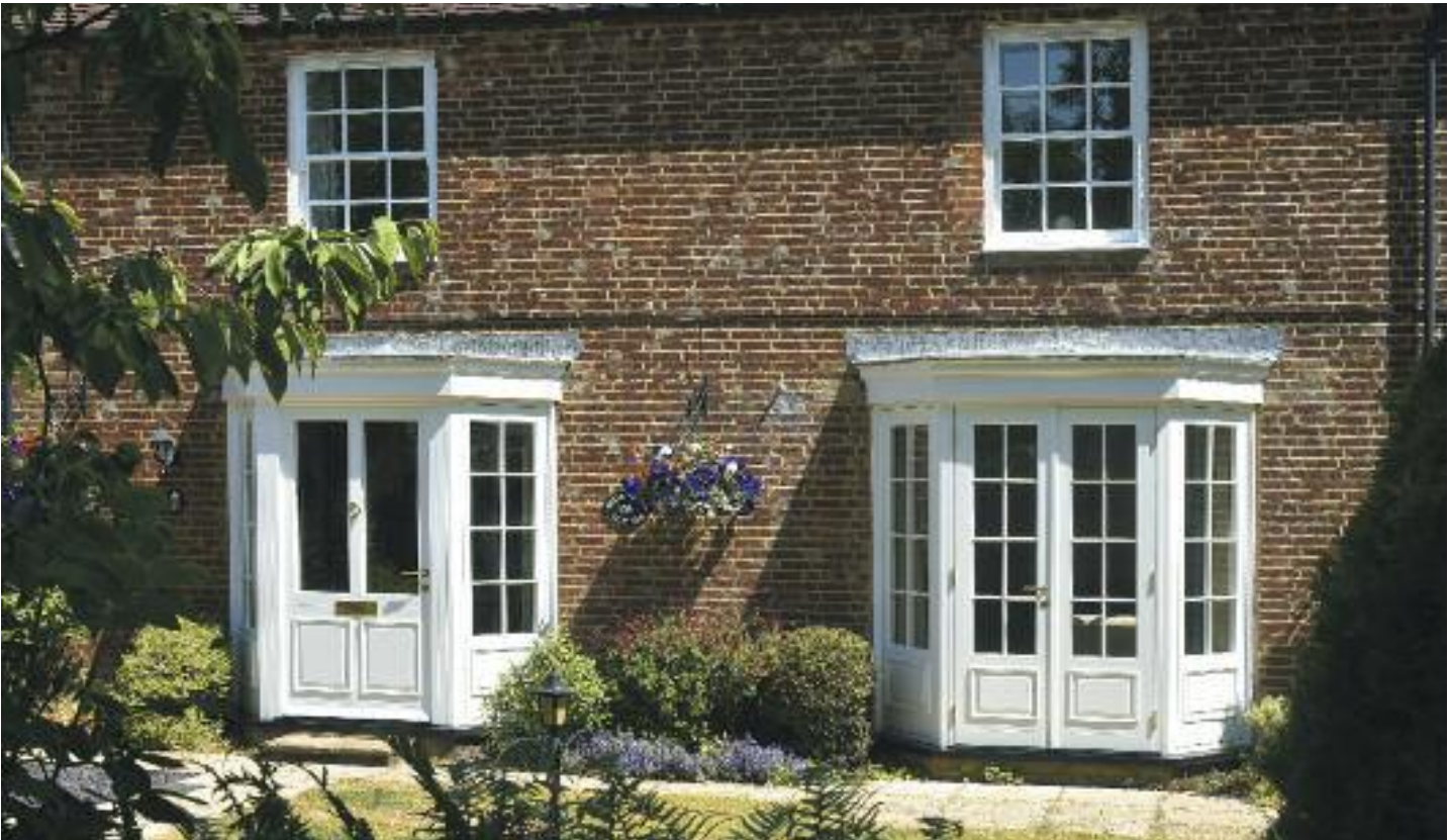
Kingston design front door finished in 'White' with 4mm single putty glazing and bolection moulding. Ironmongery from Samuel Heath includes an Extended Profile handle, Ring knocker and Medium sized letter plate in Polished Brass Unlacquered. The side window panels are also single putty glazed and feature 22mm true bars.
