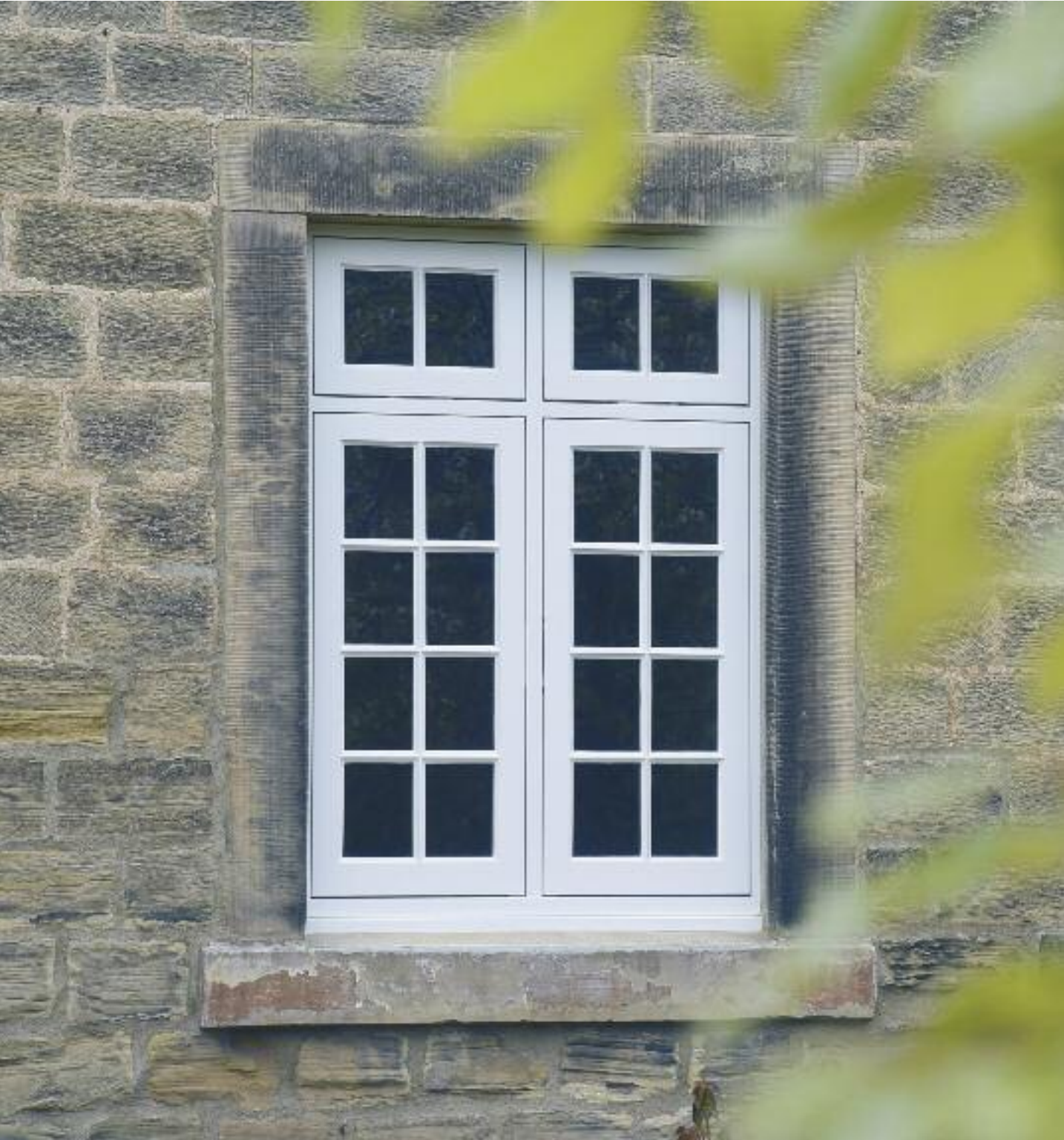
Flush casement windows finished in 'Off-White' featuring 14mm ultra-slim double-glazed units with krypton gas, along with 24mm true bars and putty glazing.
