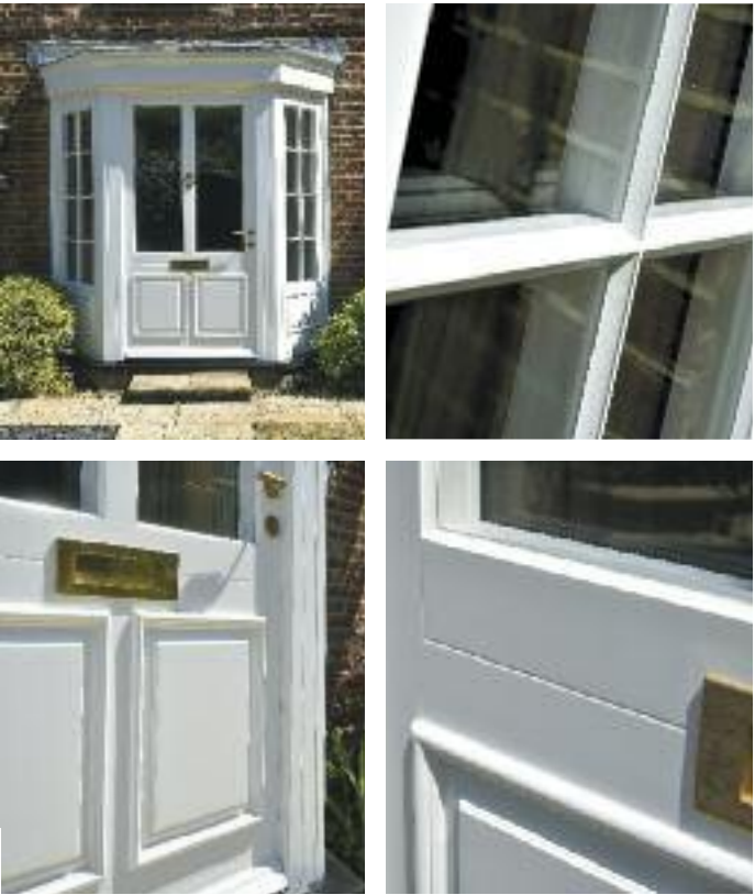
Kingston design front door finished in 'White' with 4mm single putty glazing and bolection moulding. Ironmongery from Samuel Heath includes an Extended Profile handle, Ring knocker and Medium sized letter plate in Polished Brass Unlacquered. The side window panels are also single putty glazed and feature 22mm true bars.
